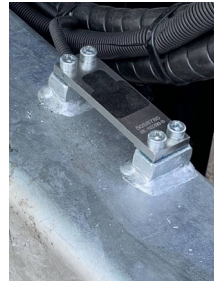
Fig. 11 – Weld plates and screw connection (detail)
